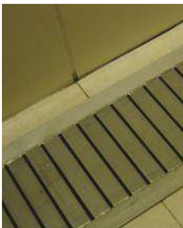
Figure 5-11: Preferred design of gratings
