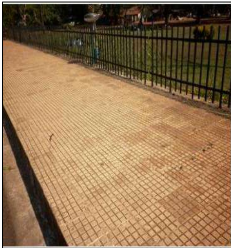
Figure 5-1: Chequered tile on footpath
