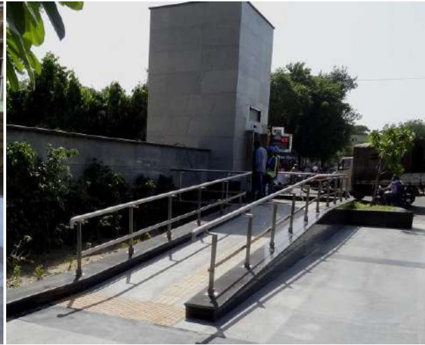
Figure 11-5: Lift access to subway crossing
