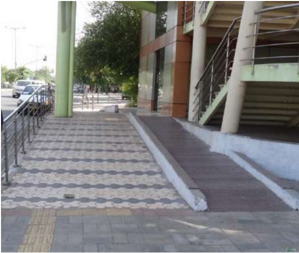
Figure 11-6: Lift access to Foot Over Bridge
