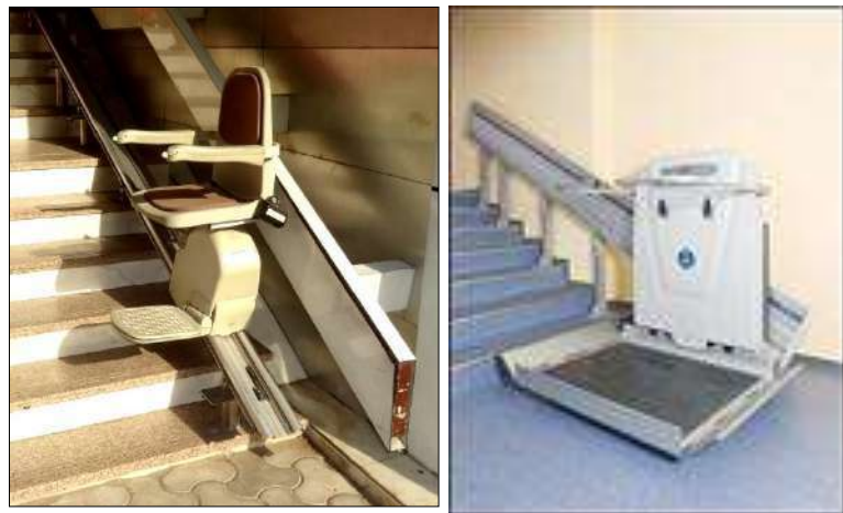
Figure 7-18: Platform chair lift and platform lift
